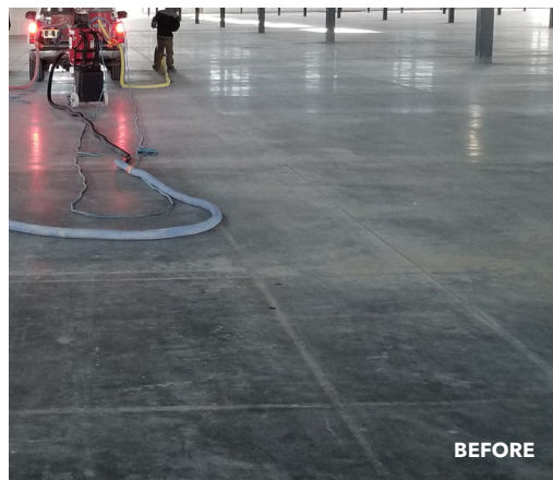
The All West Surface Prep team cuts control joints into the facility's 250,000 ft² of concrete floors. This photo was taken prior to any grinding or densification work.
